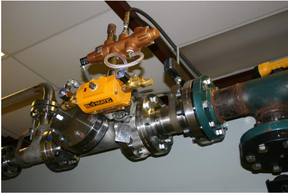
Figure D.1. Fast valve installed in BAM6QT bleed line
