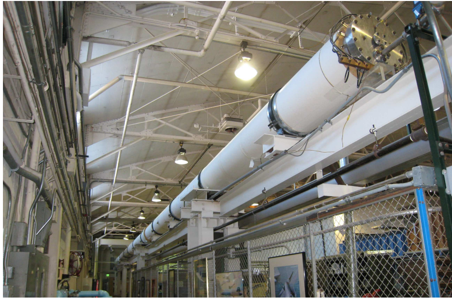
Figure 2.2. View of driver tube from the main building bay.
