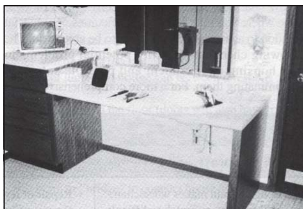
Figure 3. A lowered roll-under countertop in the bathroom provides easy access to sink and mirror. Note faucet placement on side of sink. A roll-away cart could also be used under the counter for additional accessible storage for toiletries, make-up, towels, etc.
