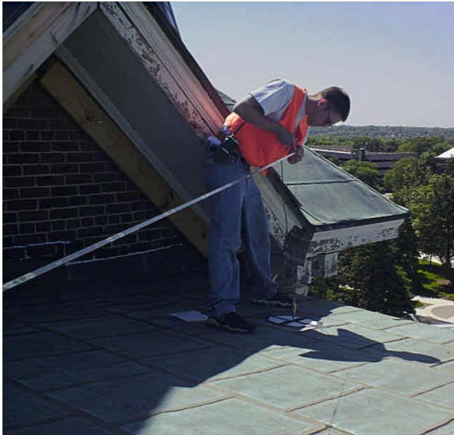
Taping to a control point
