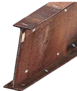
Dense Reconstruction (Point Cloud) of Steel Girder by Close Range Photogrammetry
